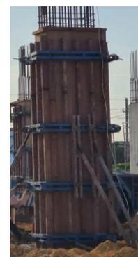
Gambar 2. Bekisting Kolom Semi-Sistem
