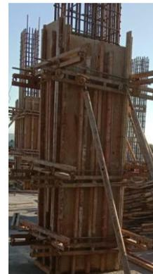
Gambar 1. Bekisting Kolom Konvensional
